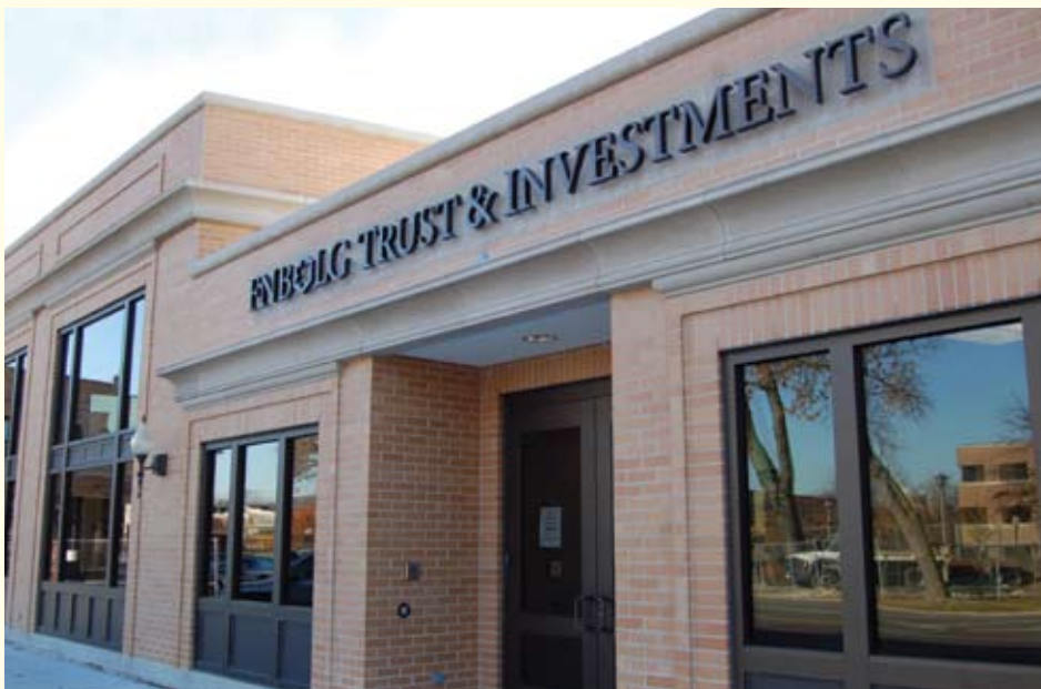
New 'Annex' building located at 600 West Burlington Avenue.
